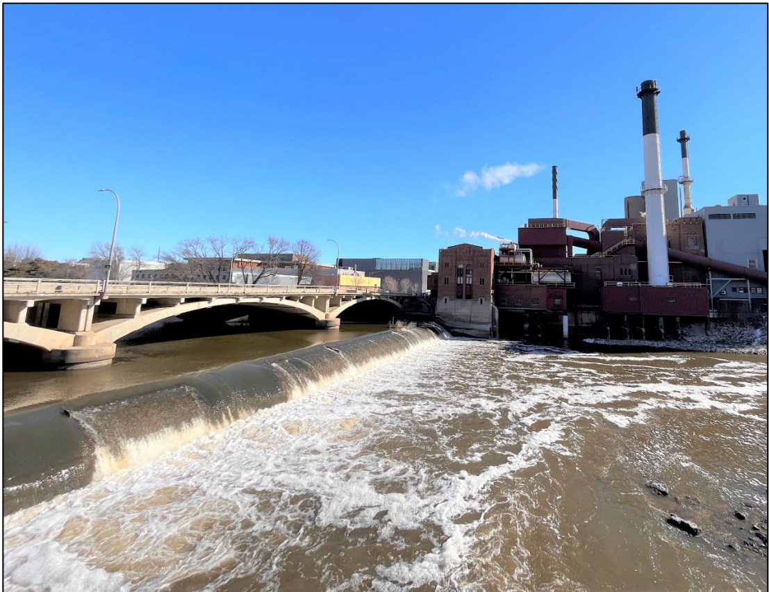
Photograph 2. Burlington Street Dam, Iowa City, IA (USACE photo).
